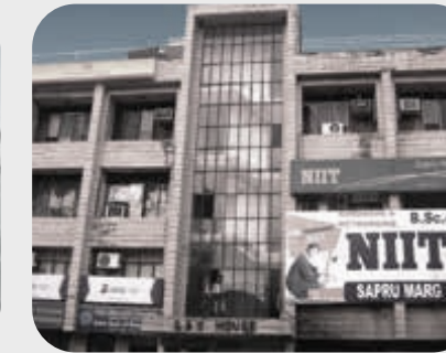
SAS HOUSE SAPRU MARG
