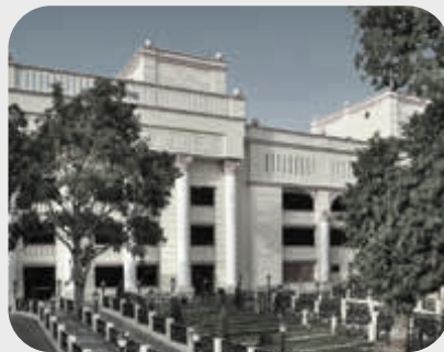
MULTILEVEL PARKING HAZRATGANJ
