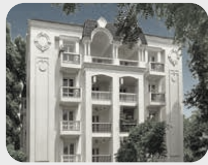
SHALIMAR ROYALE MALL AVENUE
